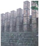
This kiln was built in 1887. This kiln was built using the slanted ground angle of 17 degrees inclination. A large size ceramic pipe fired in the Taisho era was used for the north side bank. The chimney of both ends is high, and a central chimney is low,
